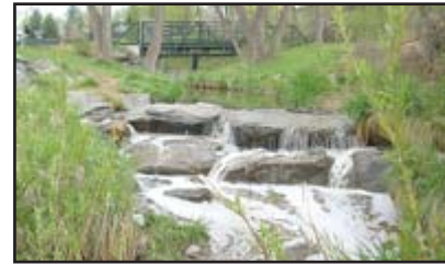
Example of simple rock dam for pond creation
