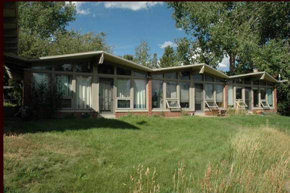
Steamboat (Hillcrest) Apartments, Architect Eugene Sternberg Nominated to the National Register of Historic Places
