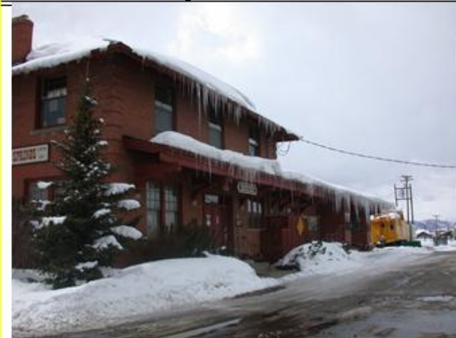
Depot roof issues
