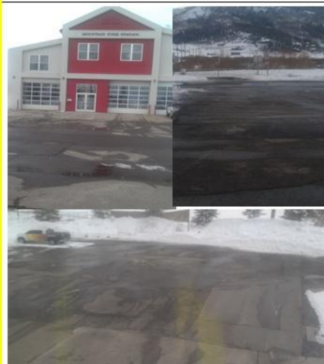
Mt Fire Station Lot and Access
