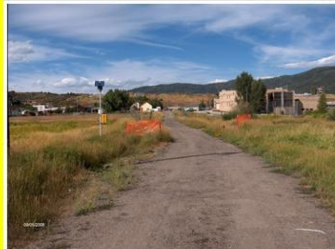
Skate Park Access Construction (Lagoon Court)
