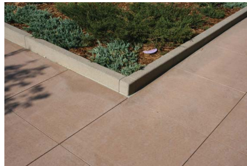
10 Concrete Planter Curb 6" x 6" Poured In Place Concrete Curb at Planting Beds In Sidewalk Standard Grey Color, Smooth Finish (See Detail)
