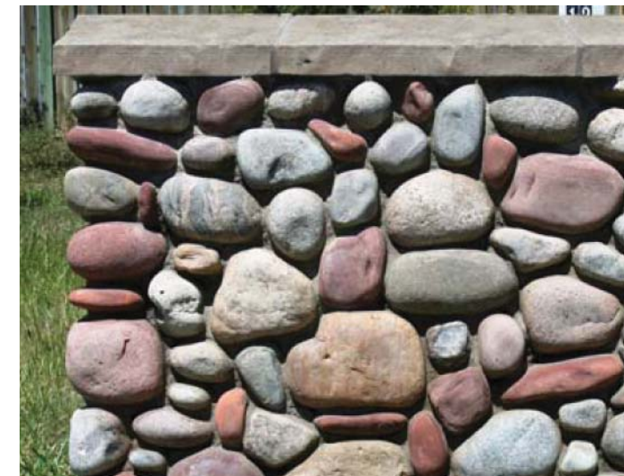
11 Seat Wall Seat Wall with Glacial Erratic Stone with Precast Concrete Cap and Recessed Wall Light (See Detail)
