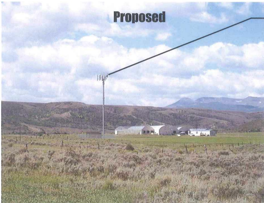
Proposed 100' Monopole with (4) AT&T Antennas Per Sector, (3) Sectors
