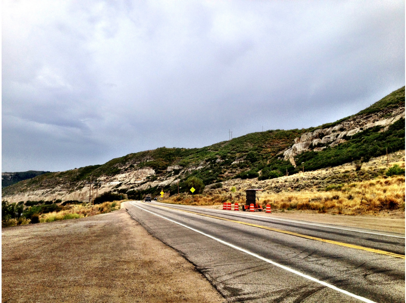
Figure 1: Looking west toward the tower site from US. Cell site is center right along ridgeline.
