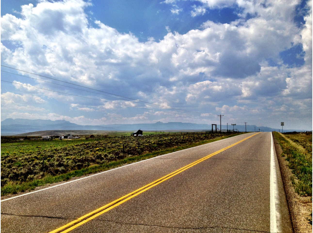
Figure 1: Looking west toward the tower site from Hwy 131 near the General Store
