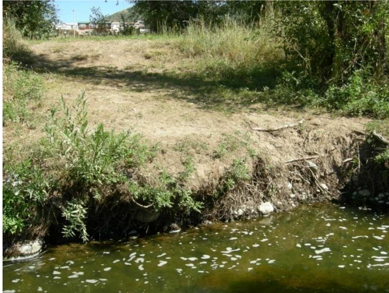
Photo 11 – Eroding Informal Access Point
