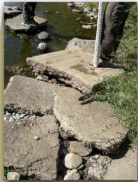
Concrete rubble in channel creates
