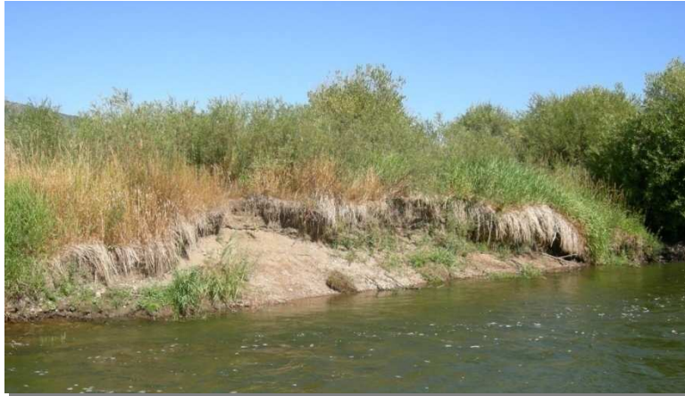
Photo 1- Existing Bank Stabilization AOI example
