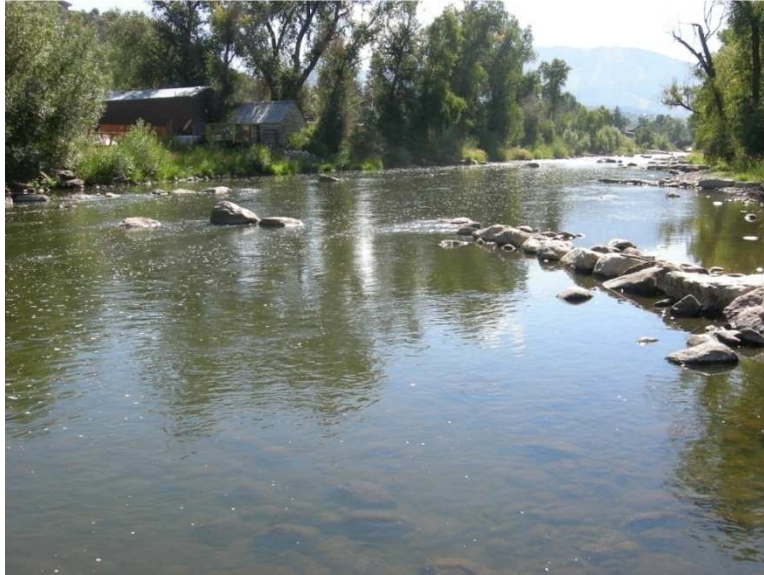
Photo 7 – Vanes have been used previously in an effort to create meanders and low flow water depths
