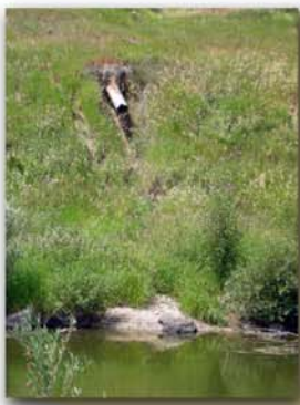
Stormwater discharge with downcutting and erosion.
