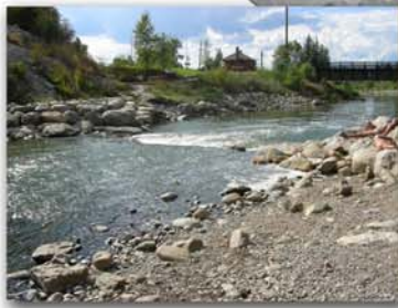
These kayak structures are of a higher quality due to rock placement, pool length
